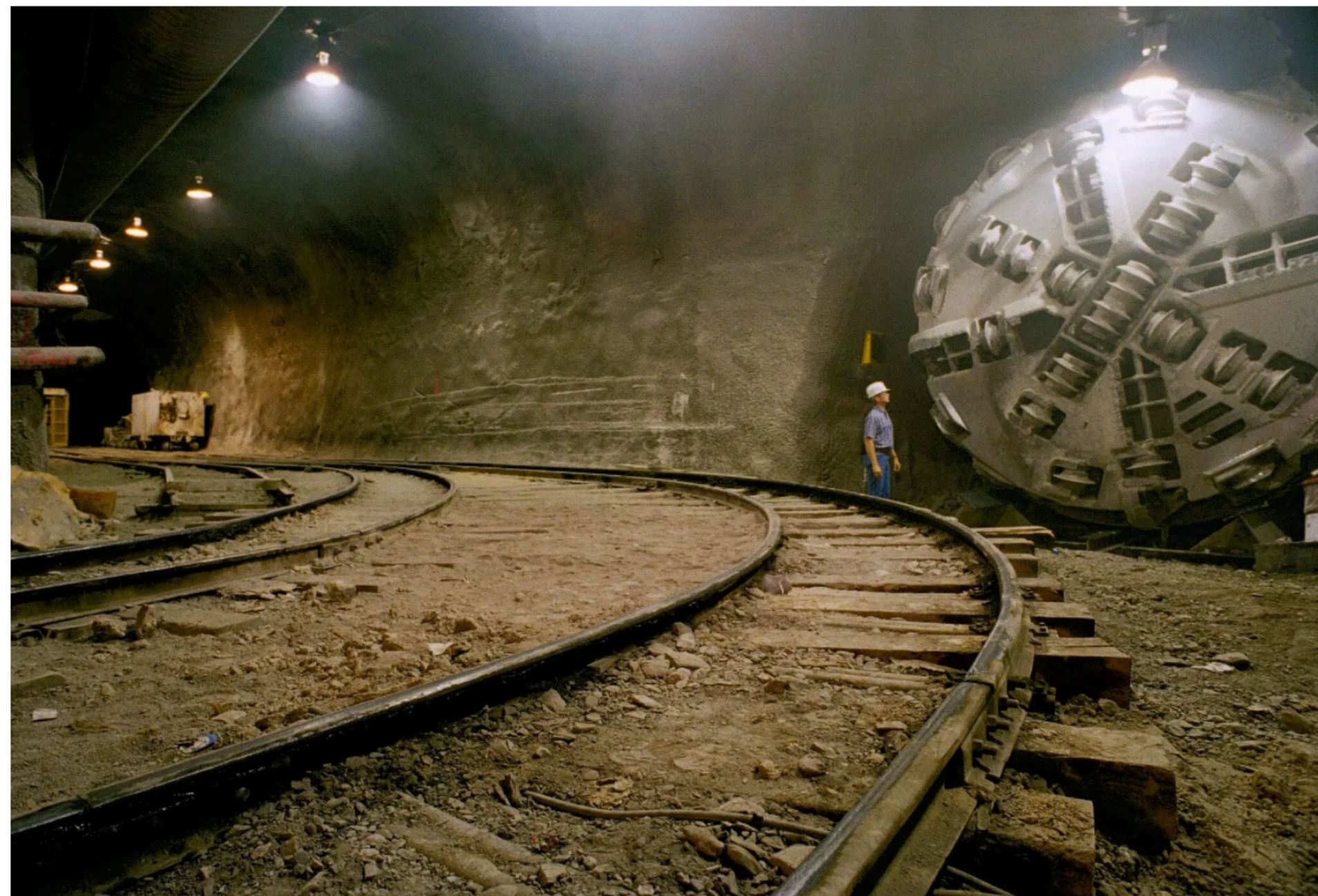
A tunnel of the Superconducting Super Collider project in 1993, which was abandoned by Congress. Ron Heflin/Associated Press
